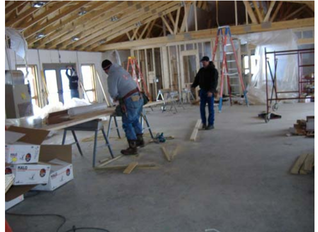
Progress continues indoors during the cold winter months.
